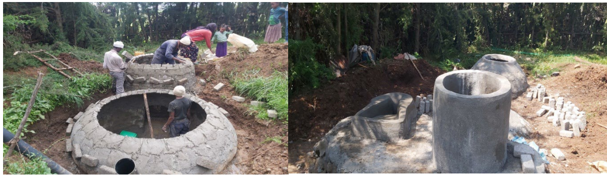
Figure 6: Biogas under construction
