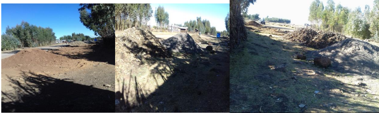
Materials supplied for completing the construction works
