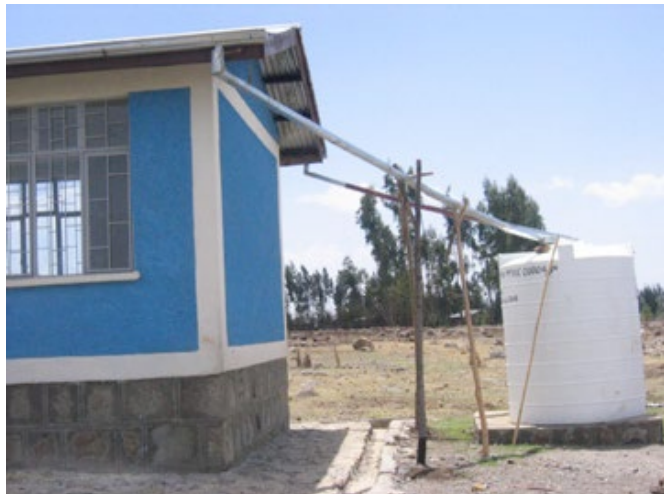
Rain-water reservoir at Workegur Primary School
